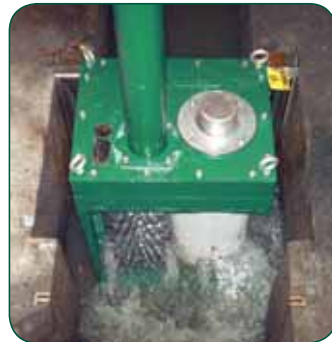
A model CMD replaced an old comminutor.
