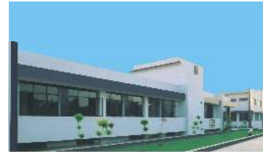
Roto Manufacturing Plant
