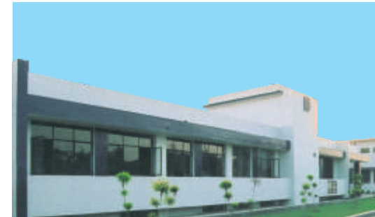
Roto Manufacturing Plant
